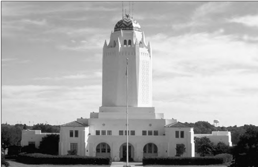
The “Taj Mahal” has been a symbol of flying training since it was built at Randolph Field in 1931. Originally constructed as the base administration building, it ingeniously enclosed a 50,000-gallon water tank.
