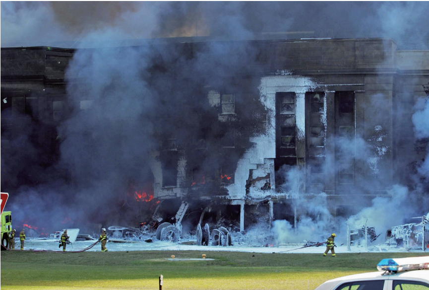
The Pentagon, minutes after the crash of American Airlines Flight 77. Foam residue is visible on the building's facade, before its collapse. Unattributed DOD photo.
