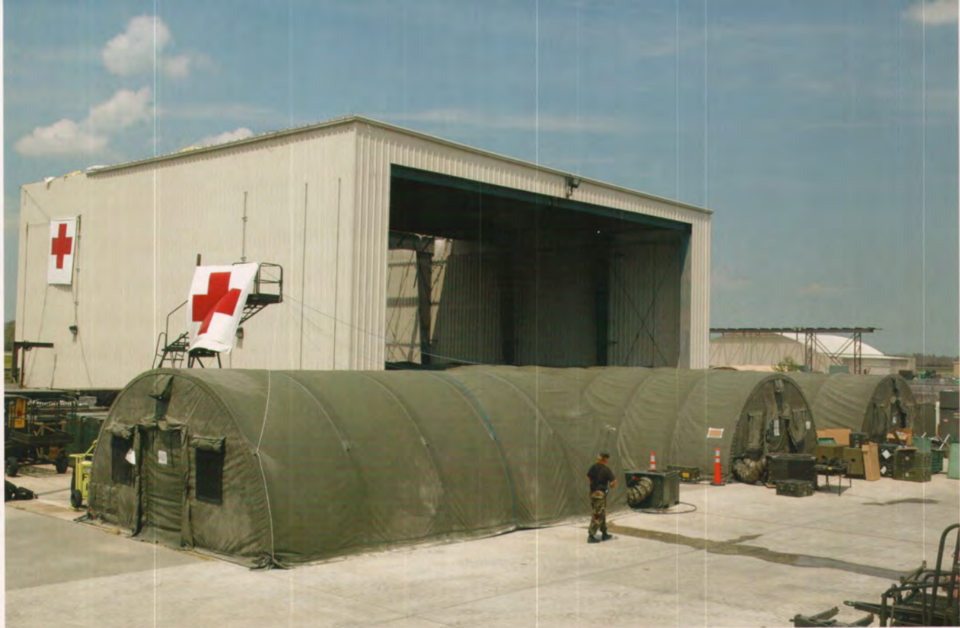
The Air Guard Expeditionary Medical Support facility at NAS New Orleans in Belle Chase, Louisiana. This facility supported thousands military personnel participating in hurricane relief operations in Louisiana. (Photograph by MSgt Bob Haskell)
