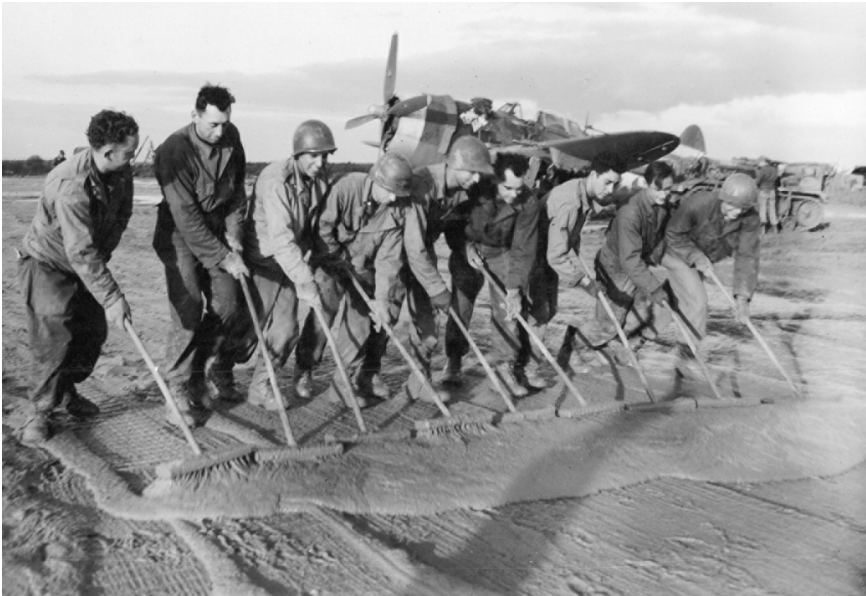
Aviation Engineers Clear a Runway. February 1945 brought rain instead of the snow that dominated most of the previous month. Here, First Tactical Air Force (Provisional) engineers clear mud off of a runway. National Archives.
