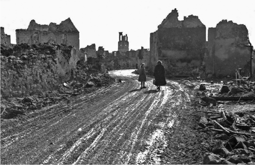
French Civilians in Mittelwihr. Artillery barrages and aerial bombardment devastated scores of Alsatian towns during the campaign to clear the Colmar Pocket. Here, French civilians survey the damage in Mittelwihr, a small town just north of Colmar, on February 8, 1945. National Archives.
