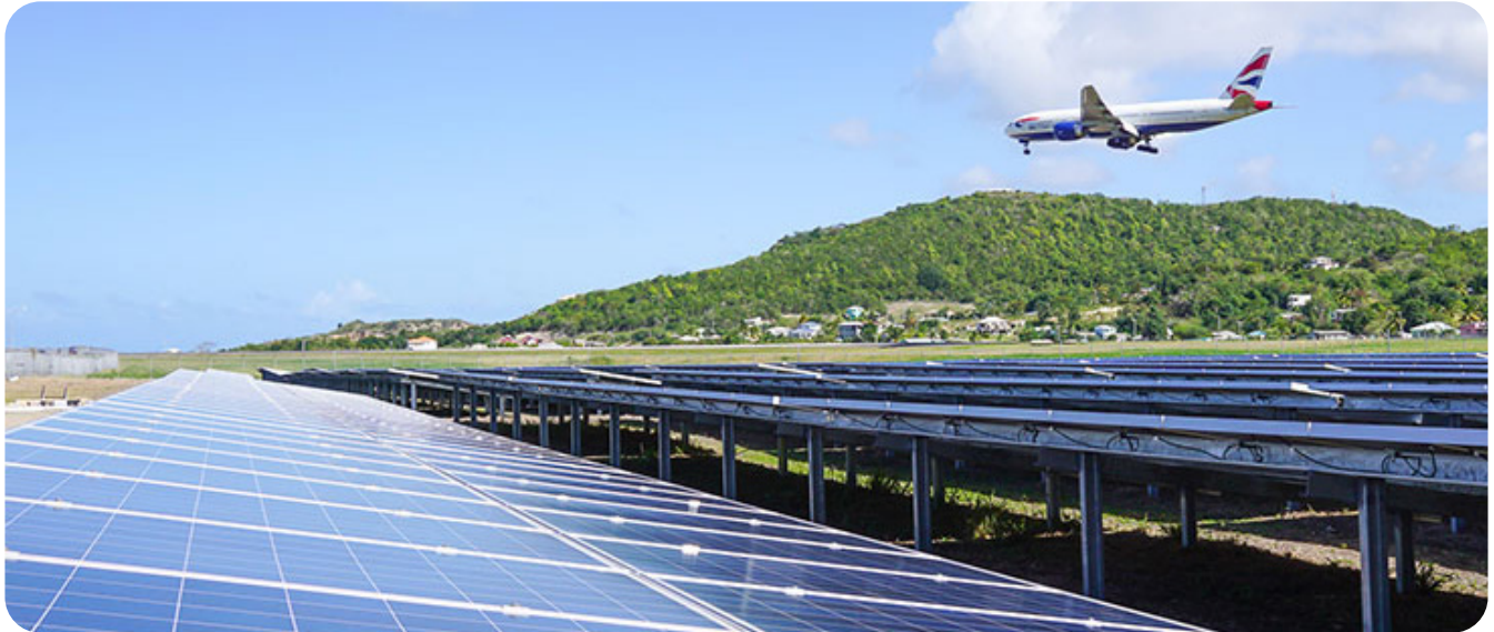
RLB Airport Solar Farm
