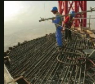
Rebar construction © Emaar Properties PJSC
