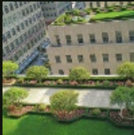
Roof garden of Rockefeller Center buildings. (Image: Wikimedia Commons)
