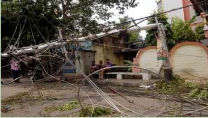
Hanging electric pole (The Hindu)
