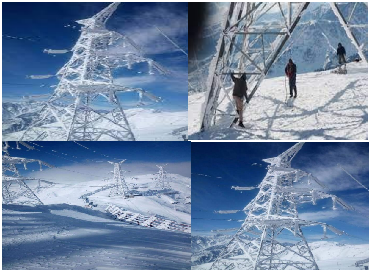
Figure 7: Impact of snowfall on Transmission lines
