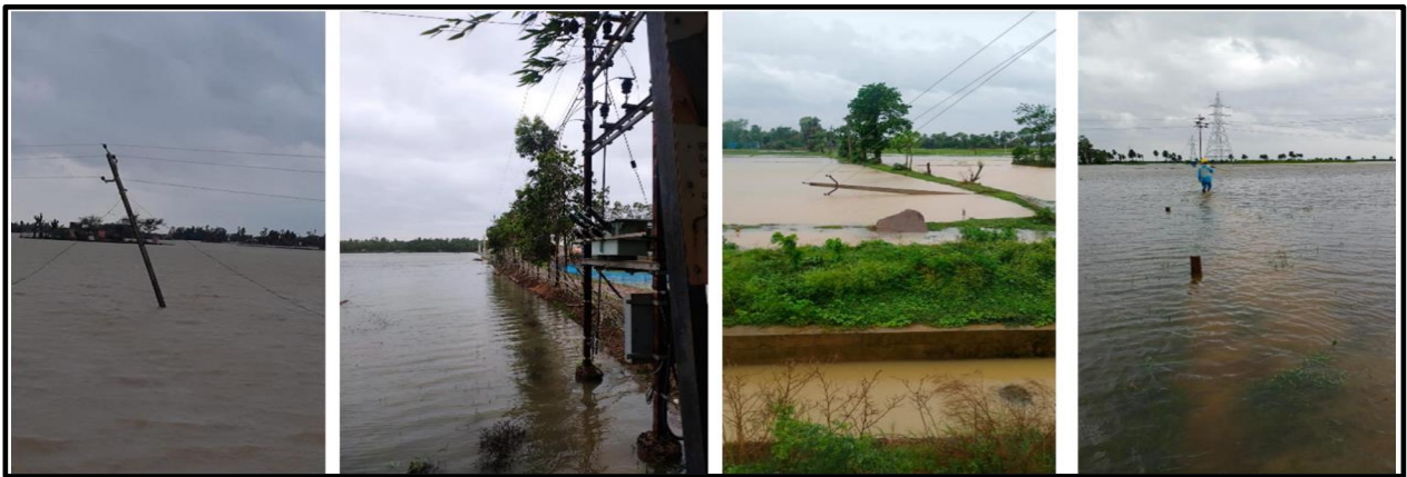
Figure 9: Impact of Cyclone on Power System
