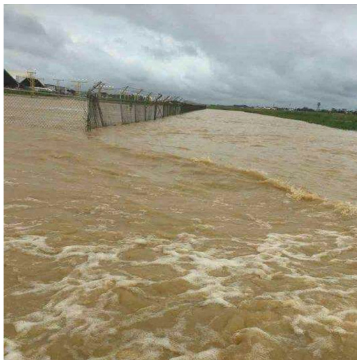
Flooding of the Piarco Airport (Trinidad and Tobago) perimeter (Photo: Kenneth Kerr)
