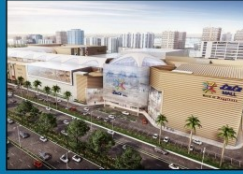
LULU MALL LUCKNOW
