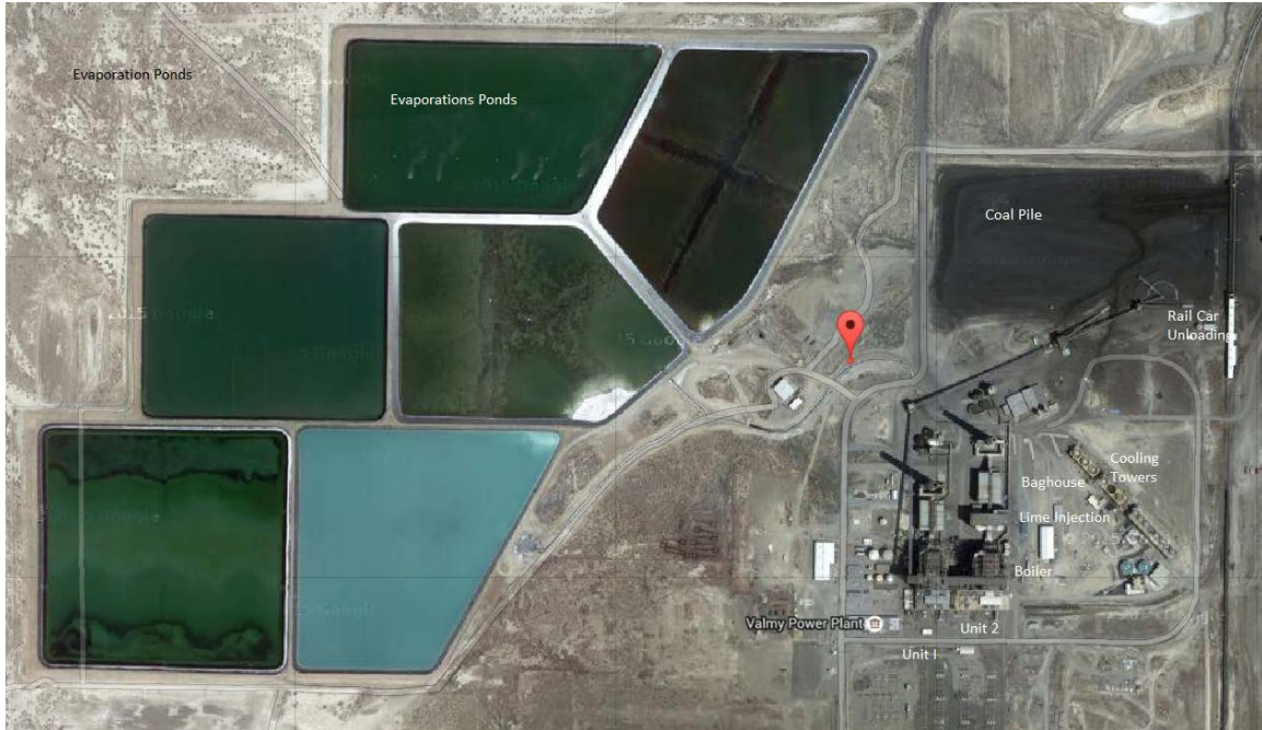
Figure 6. North Valmy power plant layout as shown from Google Maps.
