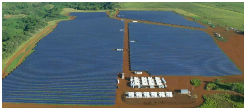
Figure 11. Tesla solar-storage facility in Kaua'i
