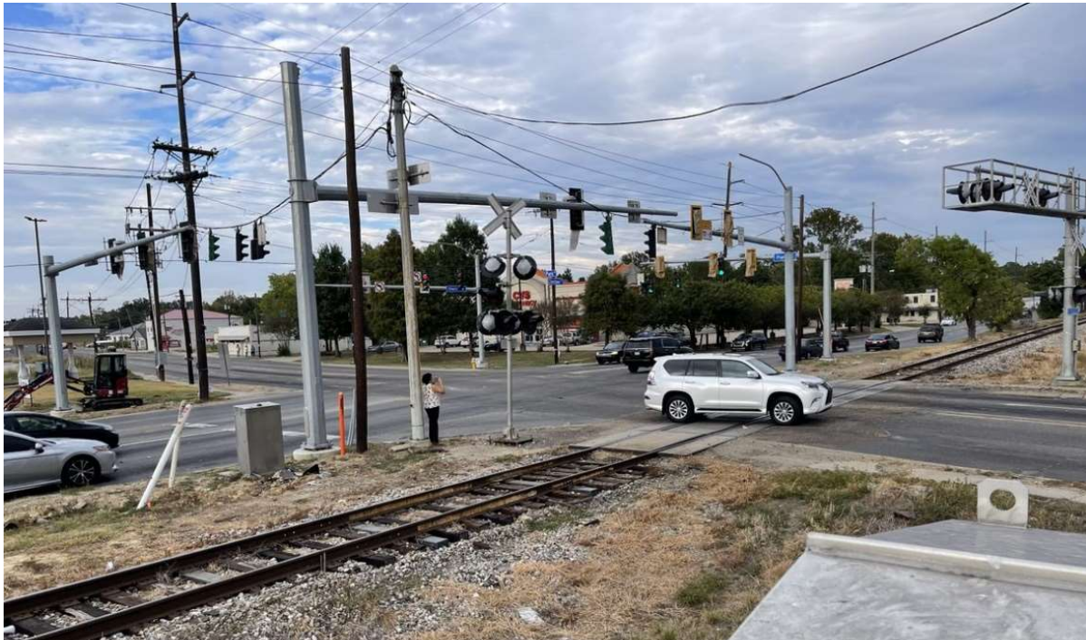
Figure 22: The grade crossing at LA 67 and Choctaw Drive in Baton Rouge is ranked first in Louisiana in terms of collision frequency
