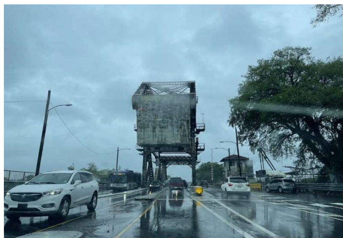
Figure 60: St. Claude Moveable Bridge
