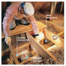
Fold the bag and stuff it into the open stud cavity. Add more insulation to the bag if it doesn't fit tightly. Plug all open stud spaces, then cover the soffit (photo 3, Page 1.7).
