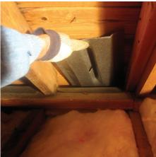
Place rafter vents in between the rafters where the ceiling meets the floor. Photo courtesy of Doug Anderson
