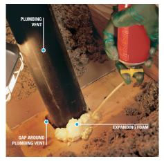
If the space around your plumbing pipe is wider than 3 inches, you may need to stuff some fiberglass insulation into the space to serve as a backer for the expanding foam. Once the fiberglass insulation is in place, follow the directions on the can to foam the space around the pipe.
