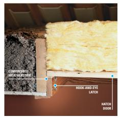
Attach hook-and-eye fasteners to the attic door and stops. Position the eyes so that the weatherstrip is compressed when you latch the hooks.
