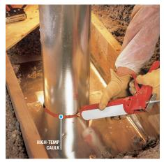
Seal the gap between the flue and metal flashing with special high-temperature caulk. Don't use spray foam.
