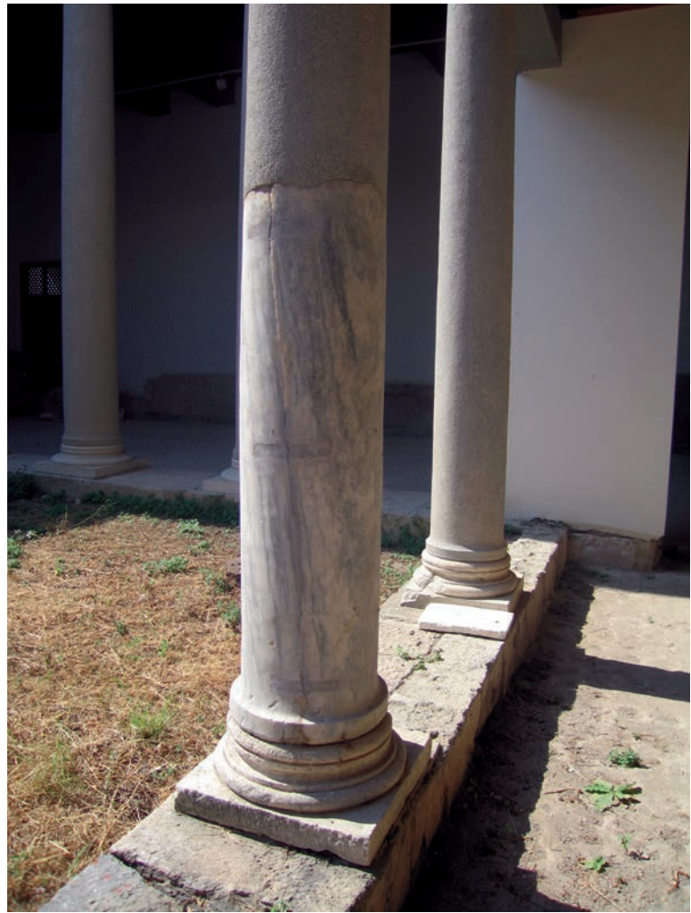
Fig. 1. Kos, Casa Romana. Column drum from cipollino nero in room XXVIII, incorporated in the restored column (A.'s photo).
