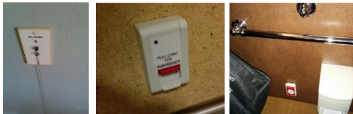
Figure 4.4. Wall sensors in 3 different communities. Two pull cords (left and middle) and a button (right)
