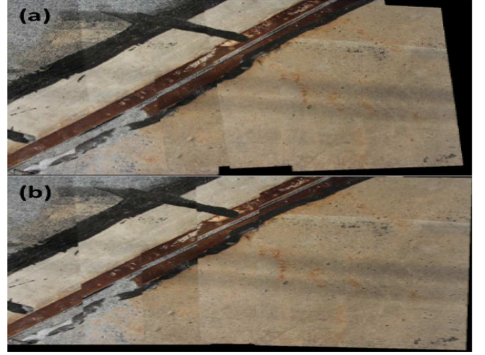
Fig. 11. Stitched images before and after distortion suppression. (a) Stitched images obtained by minimizing the misalignment of matched points. (b) Stitched images with homography distortion removed by adding a distortion term to the optimization problem. There are eight images stitched together in this figure.
