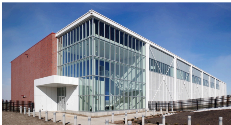
Illinois Petascale Computing Facility
