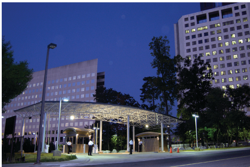
The NRC headquarters complex is located in Rockville, MD.
