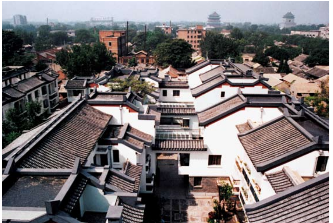
北京市菊儿胡同危旧房改造试点工程获亚洲建筑师协会金奖，并获联合国颁发的世界人居奖 The Rehabilitation of Beijing and New Courtyard House Complex Development Project at Ju'er Hutong won the Gold Medal for Architecture from ARCASIA (Architects Regional Council Asia) in 1992 and the World Habitat Award from the United Nations in 1993
