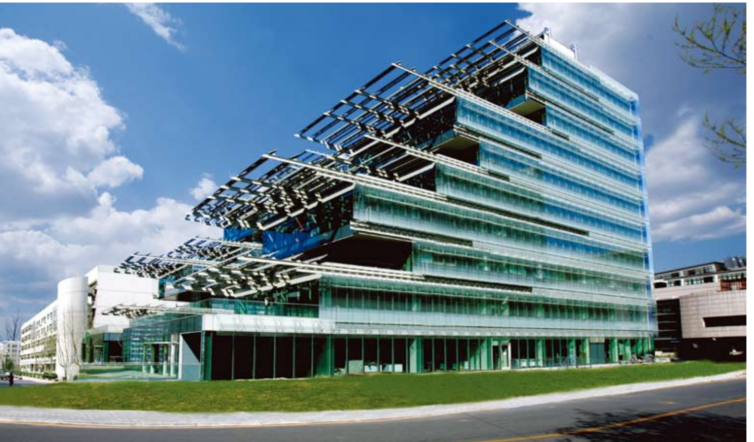
中意清华环境节能楼 Sino-Italian Environment and Energy Building
