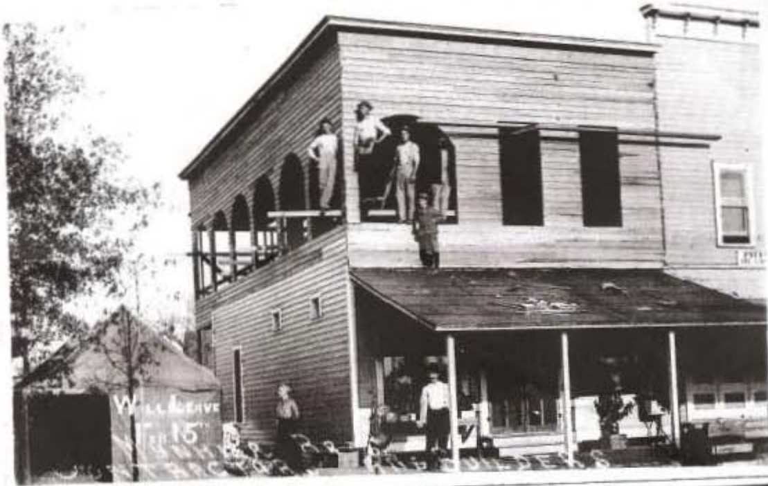
Early construction on Seventh Street East (now northbound 7 th Street) In the beginning, Seventh Street East (on the east side of railroad tracks) was considered the main thoroughfare but soon Fifth Avenue became the main street.
