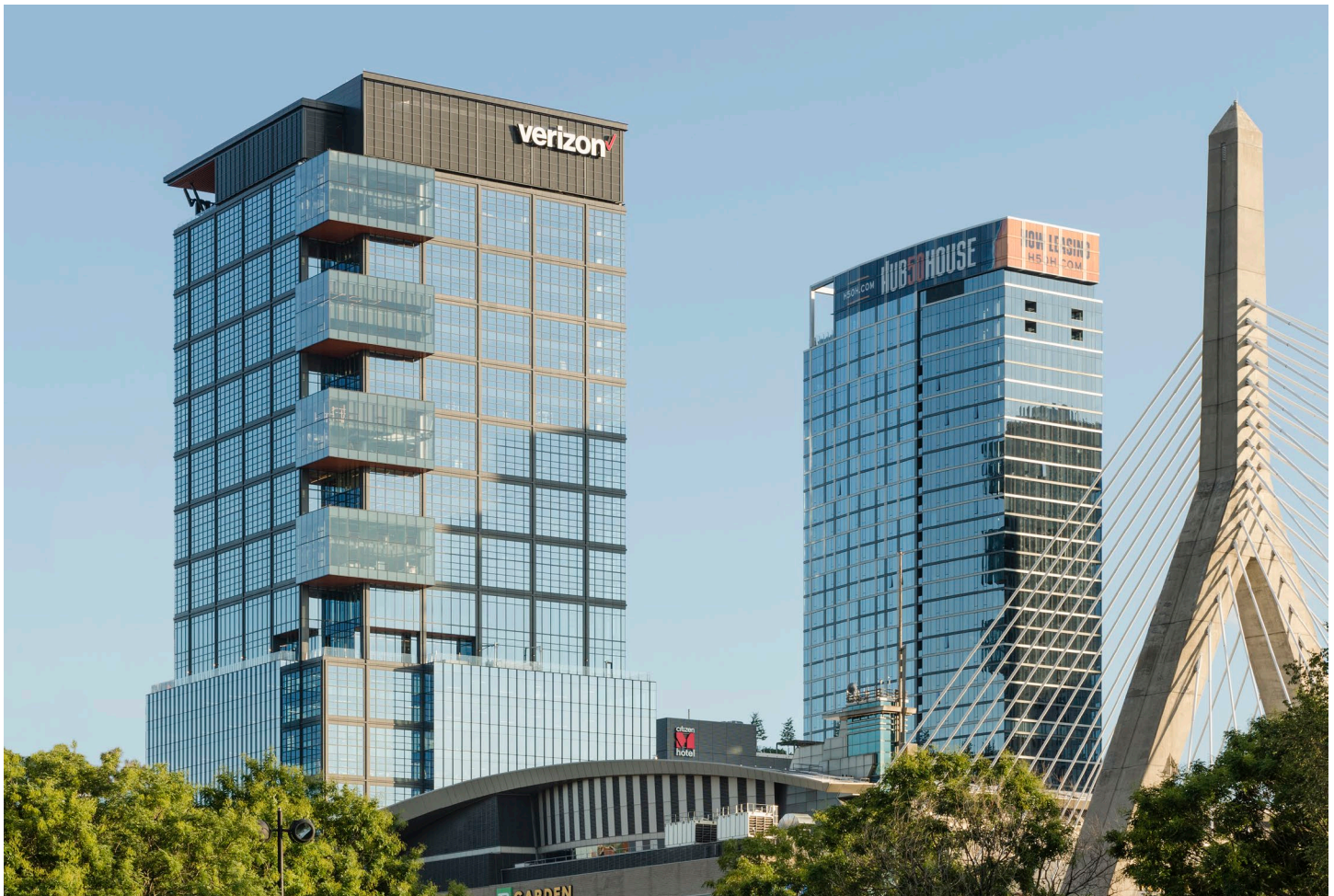
Verizon Boston Hub building (LEED Platinum certified). Photo credit: © Robert Deitchler / Gensler
