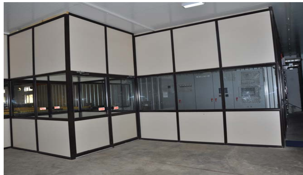
VHT Control Panel
