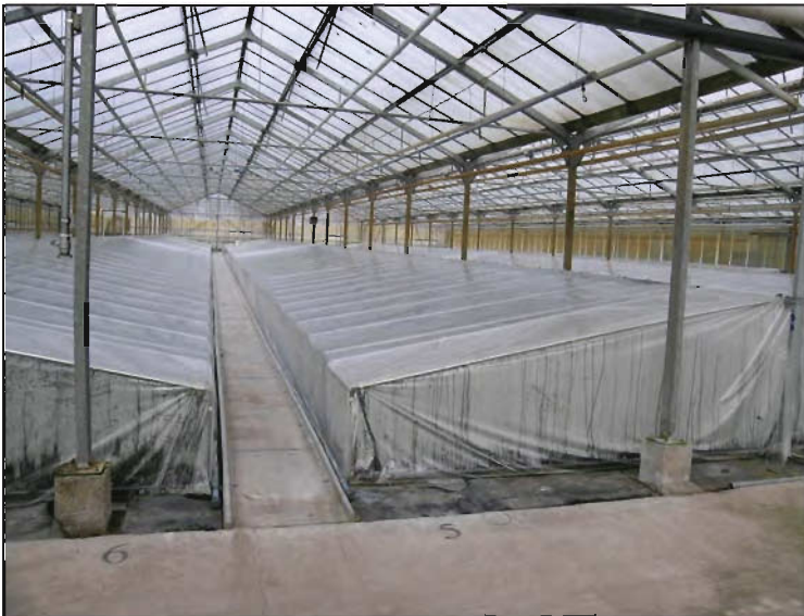
Stock plant house in Holland
