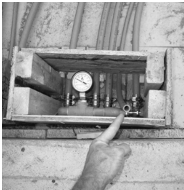
Sensor Sleeve installed in Manifold Box
