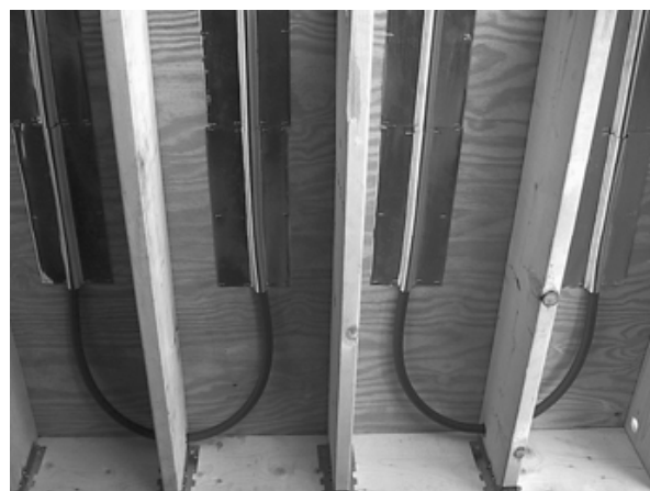
7/8" PEX in a floor Joist application
