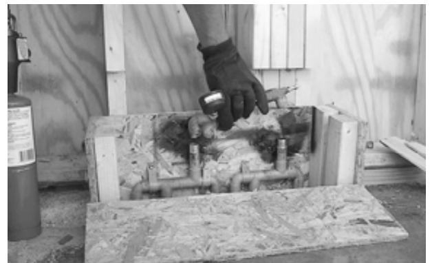
Removing the pressure testing assembly
