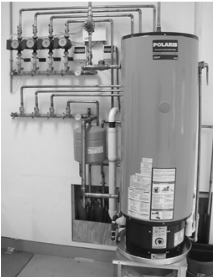
Over a mile of 7/8" PEX was installed in the floor of this state of the art dog kennel in northern Vermont. A 50 gallon, 199,000 BTU/hr., Polaris water/space heater powers a four zone open system and provides the kennel's domestic hot water.....all at 95% efficiency!
