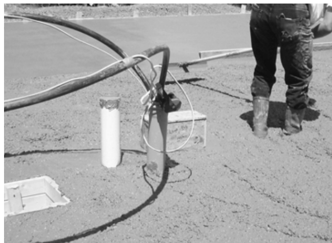
Pouring the slab around the manifold box
