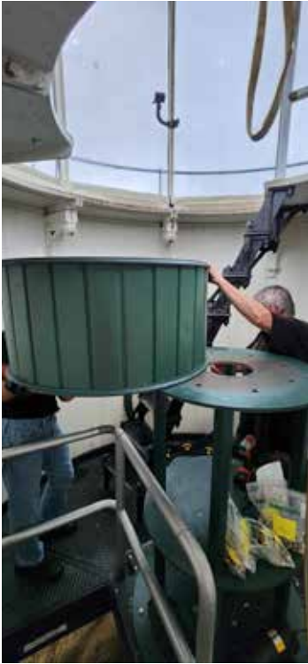
Floor cabinet assembly is maneuvered in place.
