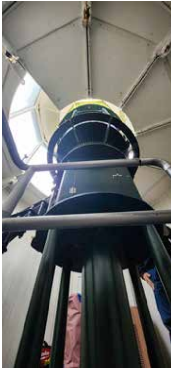
View from the bottom of the pedestal to Lantern Room catwalk.
