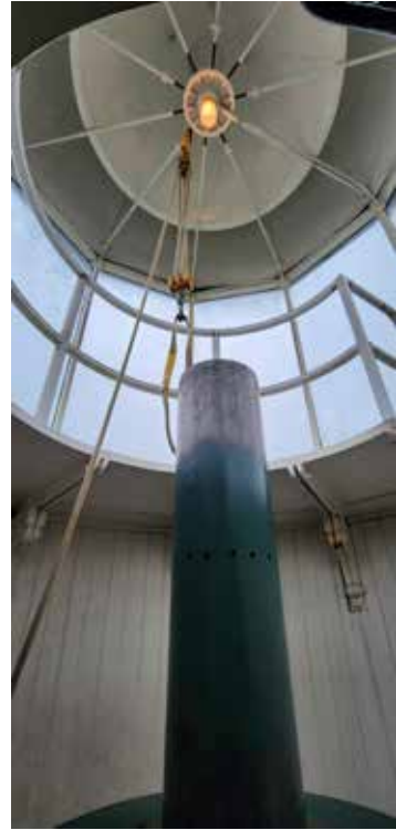
Steel column to support the rotation mechanism.
