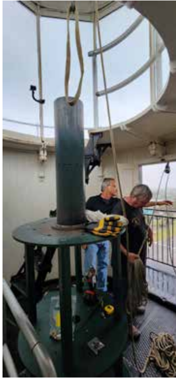
Removing the rigging used to bring the cabinet up.
