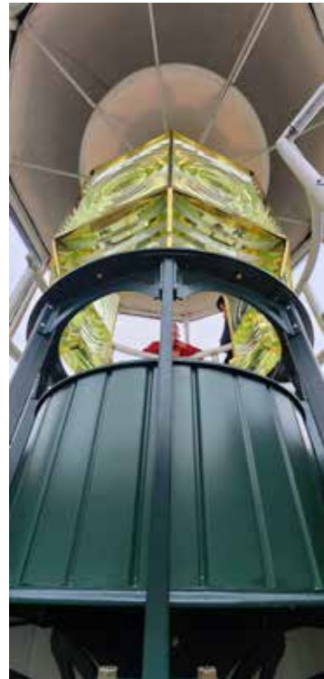
View of cabinet, fan leg assembly and lens.
