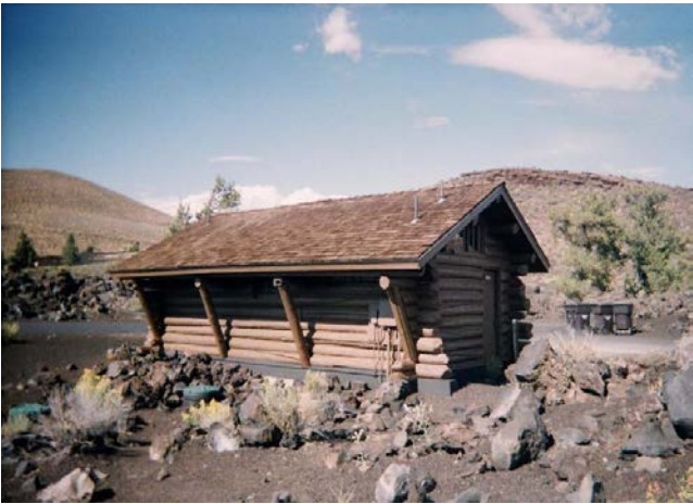
Log comfort station, 2008
