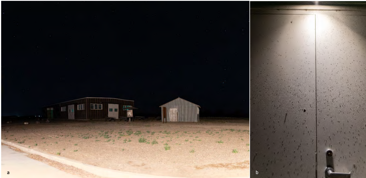
Figure 9 Light trespass across MIIN illuminating the visitor center and park grounds emanating from two facility lights which were not fully shielded (a). In addition to light trespass the lights attracted hundreds of insects (b).
