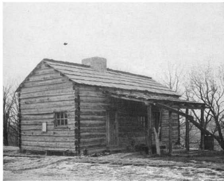
Restorations of Frontier Cabins, New Salem State Park, Illinois
