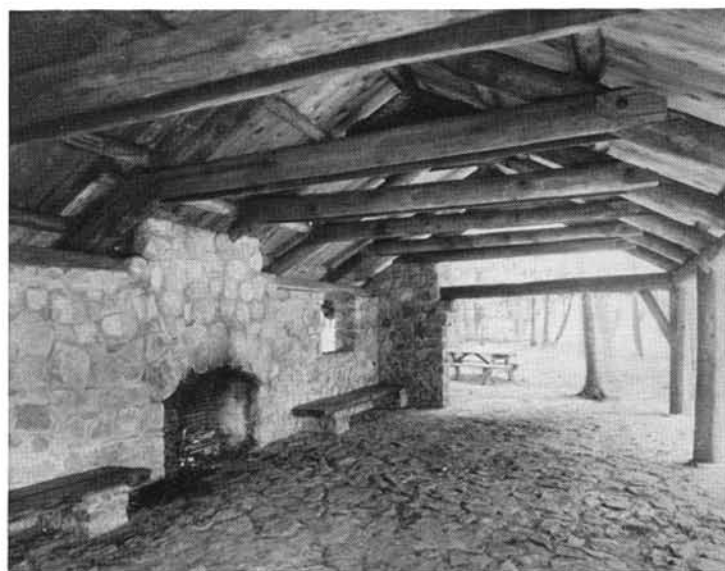
Shelter, interior view, Forest City State Park, Iowa
