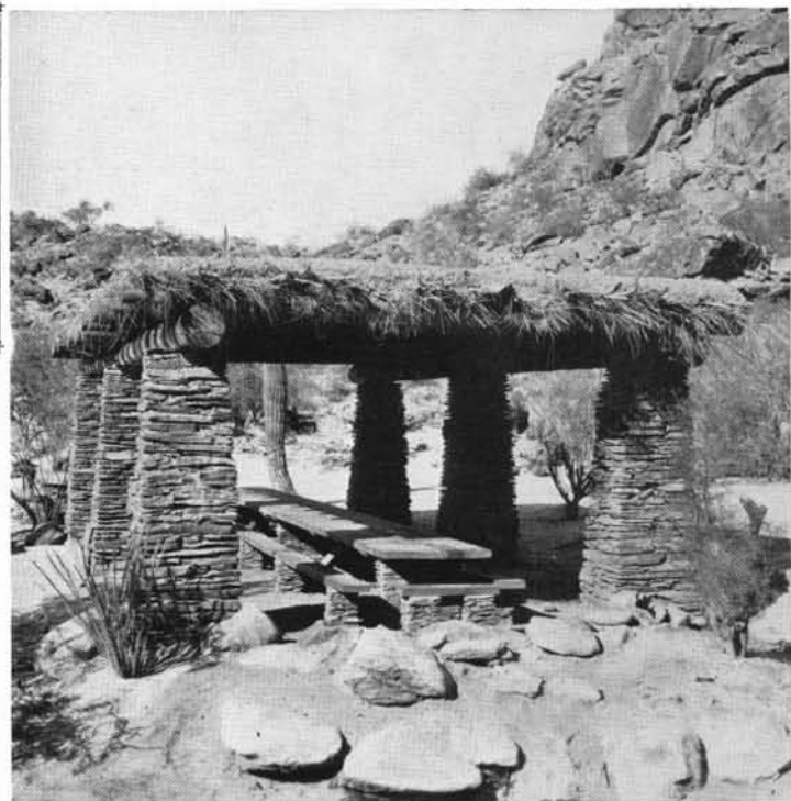
Picnic Shelter, Phoenix South Mountain Park, Arizona
