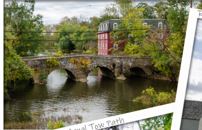
Four Arch Bridge
