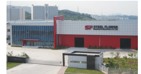
▲ Steel Processing Plant in Guangzhou, China
