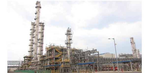
▲ Gas Processing Plant, Turkmenistan
