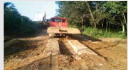
Repair of local roads
