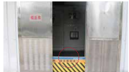
Installation of walls to protect the approach of rodents
