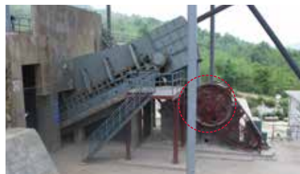
Installation of fences to prevent risks from rotating equipment
