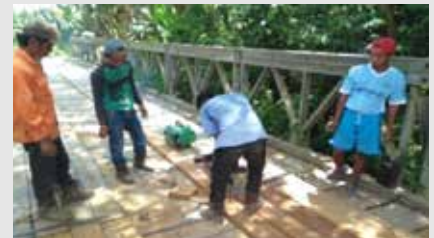
Repair of a wooden bridge in Bumi Etam Village
