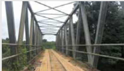
Supports for revamping a wooden bridge
