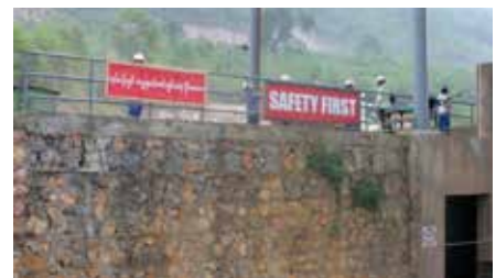
Installation of fences to prevent falling
