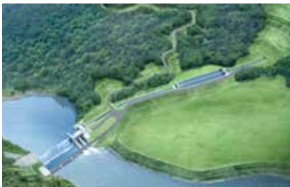
Hydroelectric Power Plant in Hasang, Indonesia
