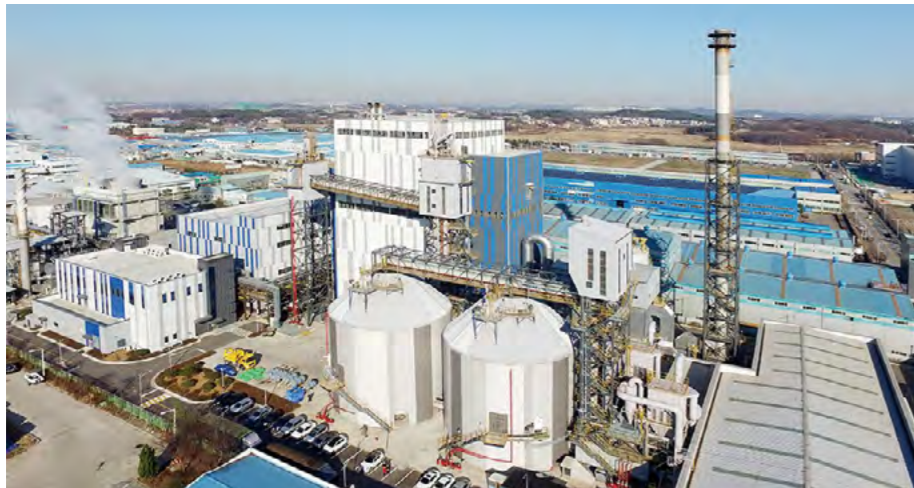
Poseung biomass plant
