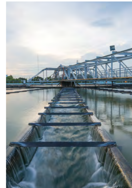
Support for Water Treatment Plant
