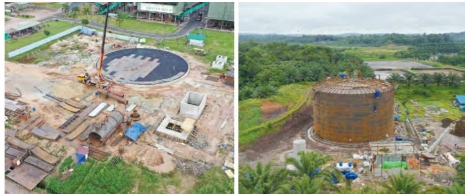
Biogas plants in PAM and TBSM (currently under construction)
