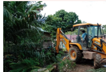
Support for entry road construction to a remote village
