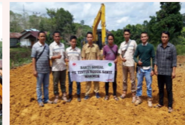
Support for earthworks for a new kindergarten
