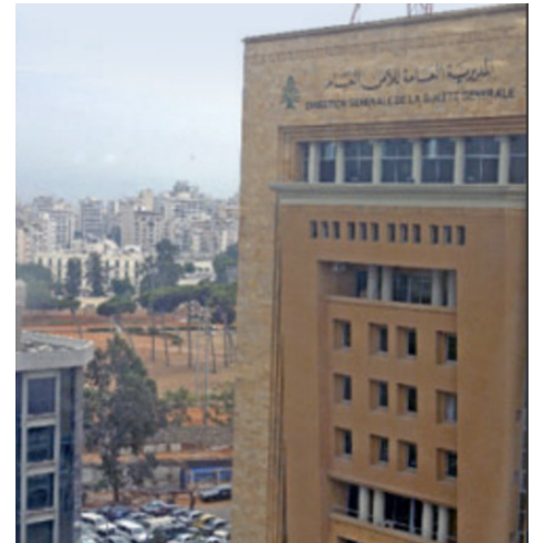
Figure 1: A picture of the GDGS building in Beirut, Lebanon from where we have located Dark Caracal operating
