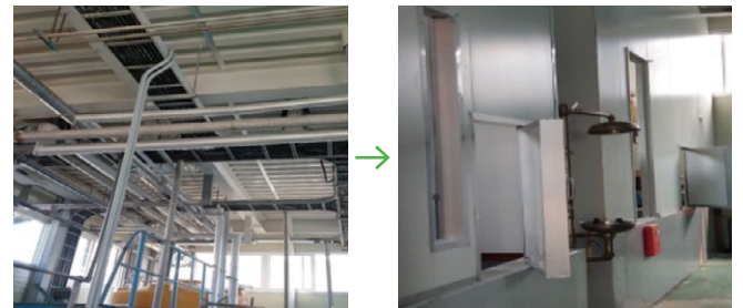
▶ Compartmentalized hydrochloric acid storage tank for wastewater treatment in Cheonan
