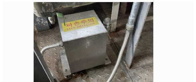
▶ Installation of a leak detector in the warm interface manufacturing room
