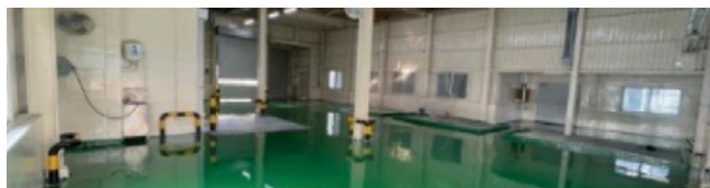
▶ Operating integrated waste storage facility at Cheongju Plant
