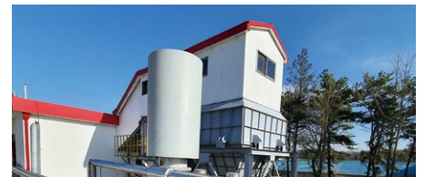
Odor masking facilities at the Yeosu Plant
