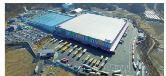
→ View of the Integrated Distribution Center in Cheonan
