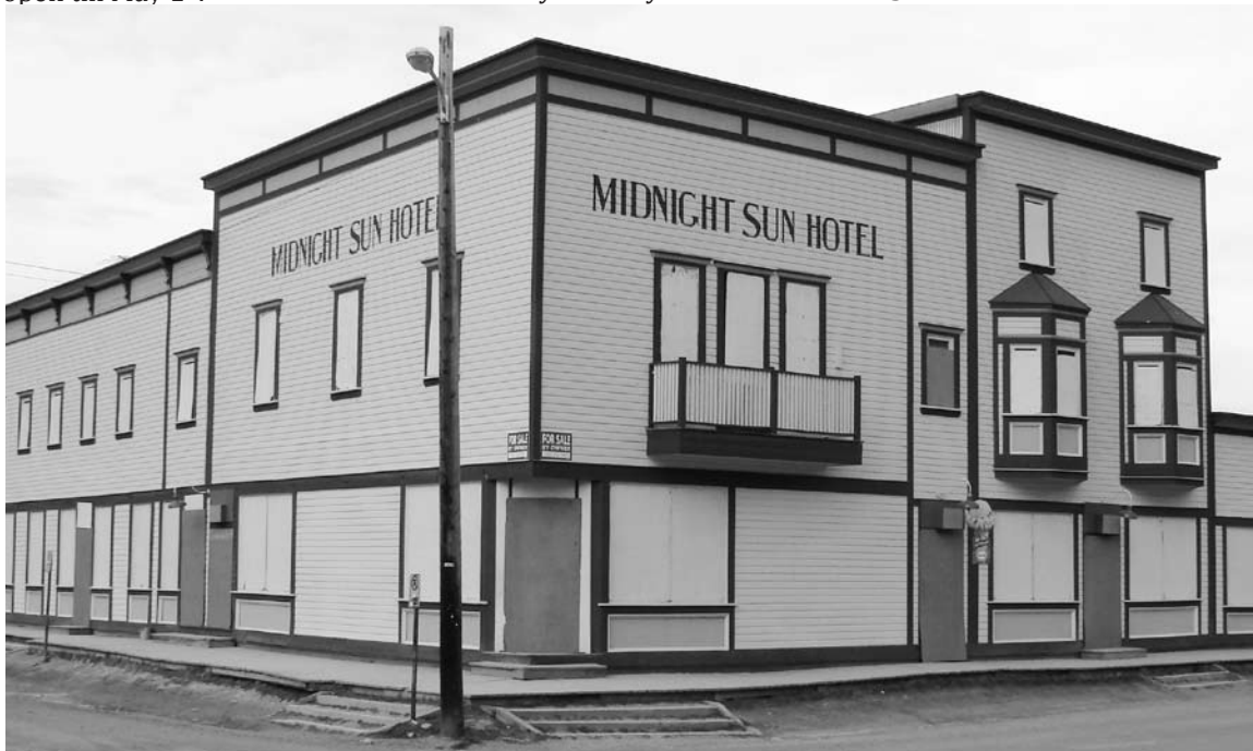
The Midnight Sun Hotel is boarded shut for the winter. Photo by Dan Davidson.
