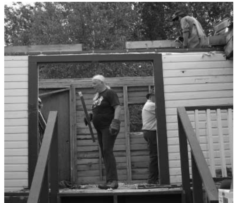
Demolition of the old entry way took place in July.
