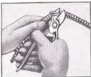
Cutter inserted between armor and conductor for cutting cable.
