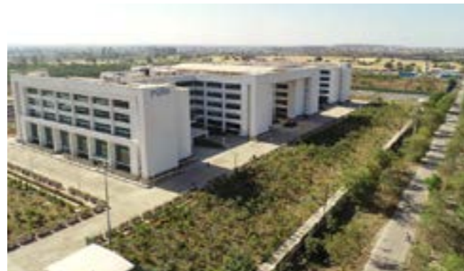
Infosys, Indore SDB – LEED Platinum certified building
