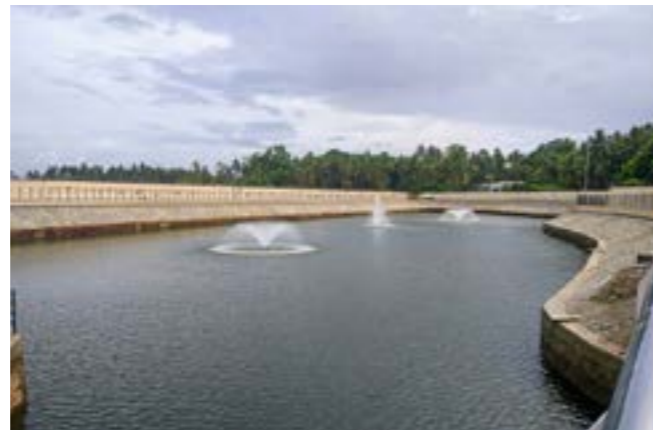
Rainwater harvesting pond in Infosys, Thiruvananthapuram campus
