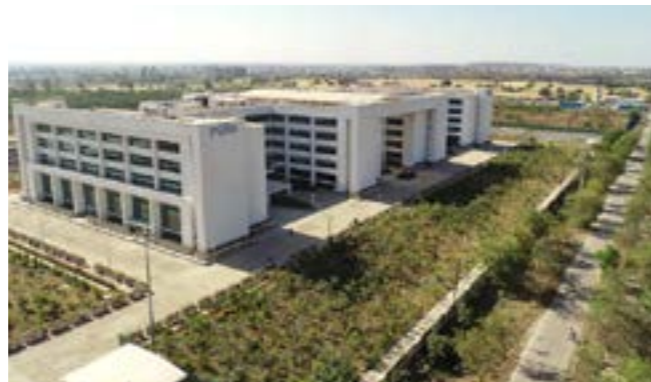
Infosys, Indore SDB – LEED Platinum certified building
