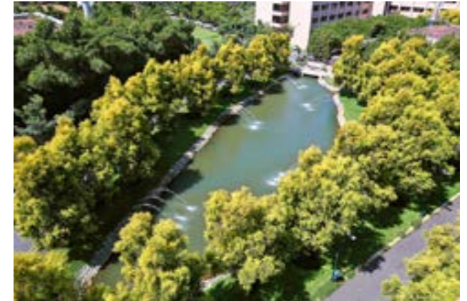
Rainwater harvesting pond in Infosys, Bengaluru campus
