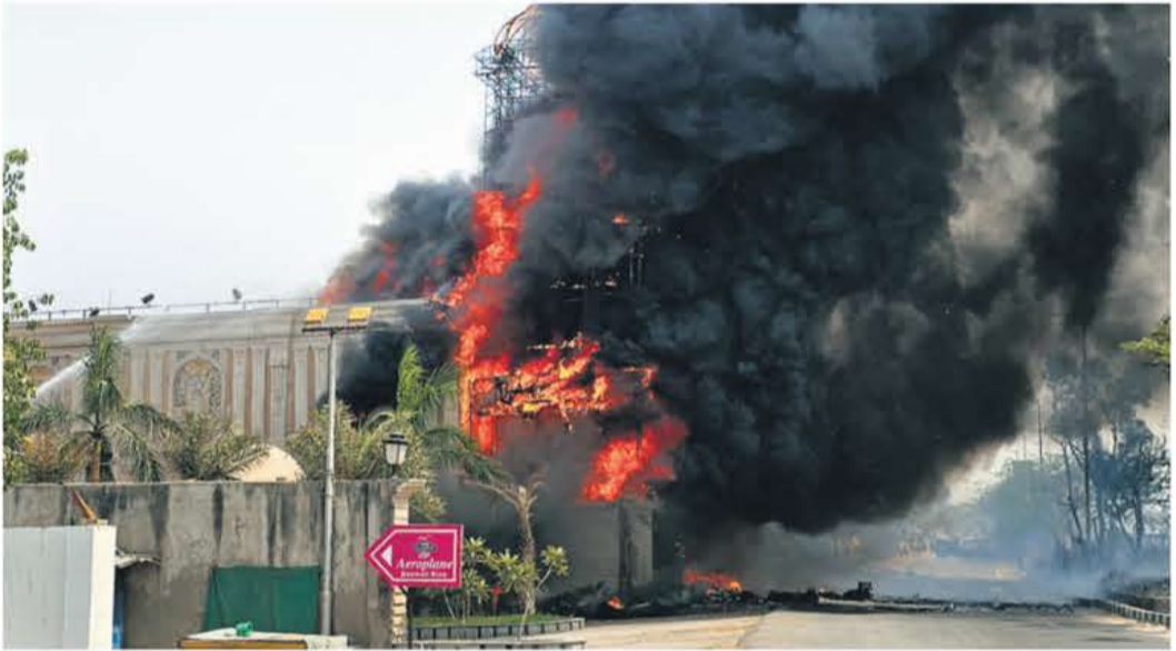
BANQUET HALL FIRE Smoke billows out after a fire broke out at a banquet hall in outer Delhi's Alipur area on Friday | PTI
