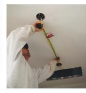
The increased circulation around the duct can dilute air quality and fool the detector. Make sure there's at least 36 in. of space between the duct and the detector.
