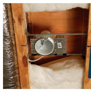
**SOLUTION** If you retrofit non-IC recessed fixtures, secure the insulation so that it cannot spring back and contact the light after it's installed.
