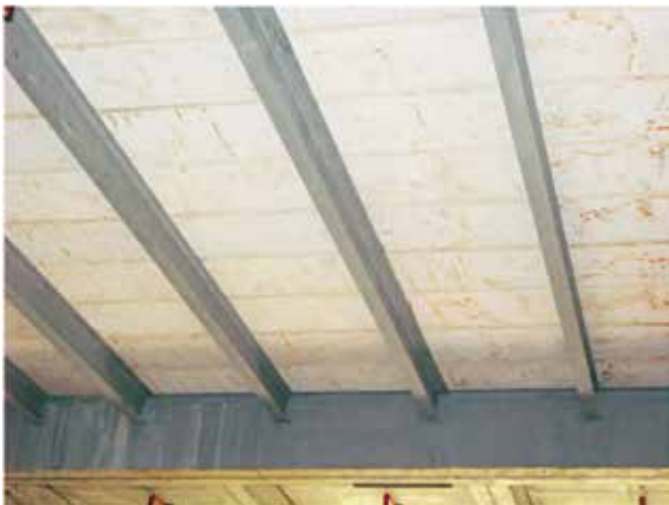
C-Type Steel Fixed with H-Type Main Beam
