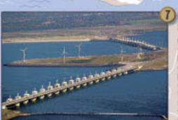
Originally envisioned as a dam, plans were completely revised, partly because of unintended environmental changes wrought by the Brouwers project. The dam would have destroyed oyster farming and decimated the fishing industry. The partially built structure was modified into a barrier with a series of giant doors that slide shut during a storm.
